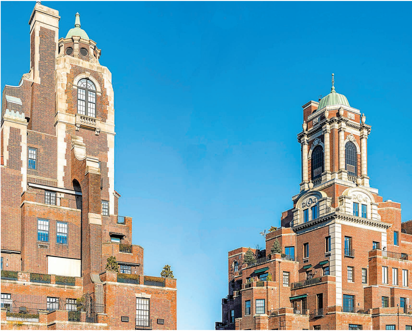
Rosario Candela's buildings at 770 and 778 Park Ave. demonstrate the terracing effect, as required by city ordinances.
